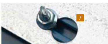
Key hole slot fixing.
