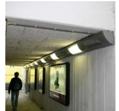
Blank infill module for continuous line mounting.
