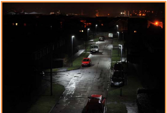
Stela LED street lighting after installation
